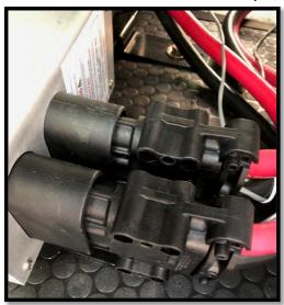
3. Correctly Installed and Fully Seated DIN Connector, Male to Female:
