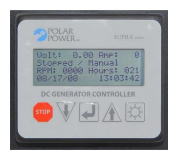
The keypad on the Supra Generator Control Panel consists of 5 buttons. Stop, Down, Enter, Up, and Back Light.
