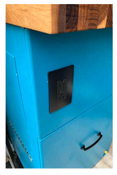
Within the kitchen cabinet is the 120VAC receptacle for inductive cooktop. Note: the inverter is 2kW pure sine wave and weighs only 16 lbs. It is located in sofa bed (not shown).
